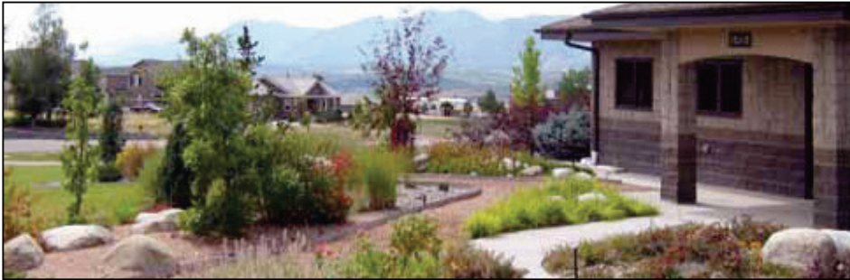
Woodmoor Water and Sanitation District's South Water Treatment Facility includes a xeriscape garden to demonstrate for customers water-saving gardening techniques.
